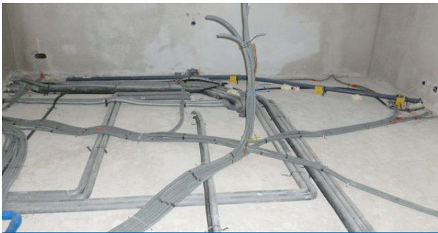
Step 1 - Basic installation Completed installation work prior to thermal insulation
