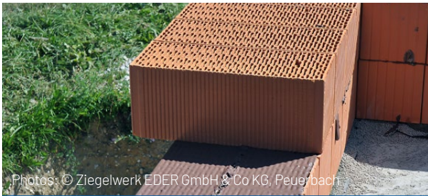
The ceiling mortar can be applied as usual after the bricks have been swept clear.
