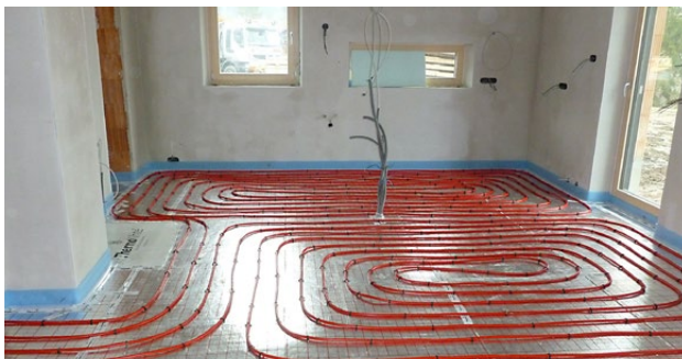
Step 6 - Installation of floor heating After the drying time of at least 48 hours
