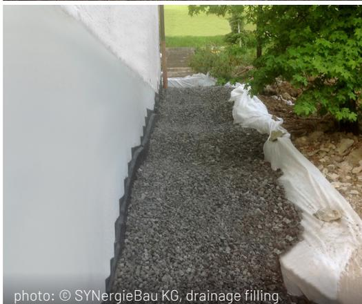
photo: © SYNergieBau KG, drainage filling
